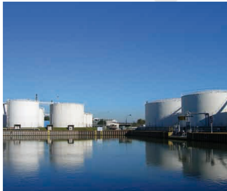
1) Storage tanks for various acids, internal coating
