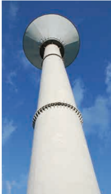
1) Water tower "Aquaglobe", internal coating
