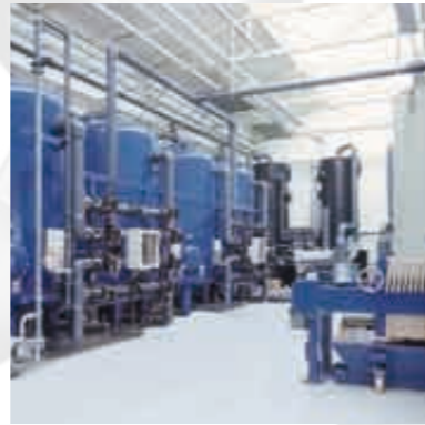
2) Sand filter vessels for drinking water, internal and external coating
