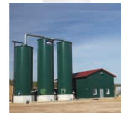
Picture: Energie-Anlagen Röring, Germany
