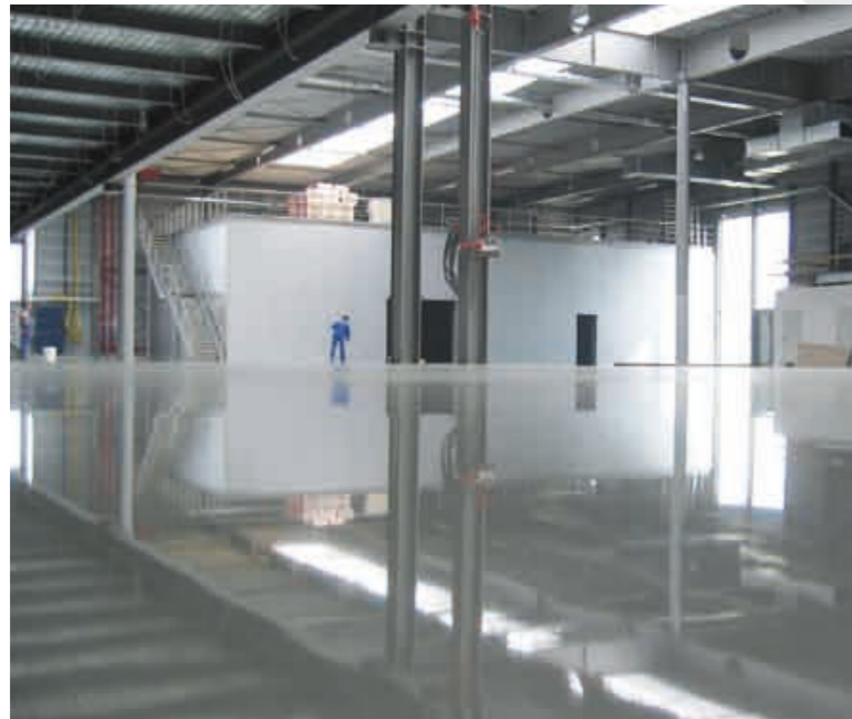
6) Storage depot, antibacterial flooring system
