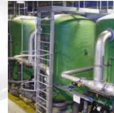
2) Drain pan for storage tanks of chemicals
