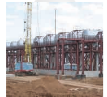
6) Crude oil separators, internal coating against SRB bacteria
