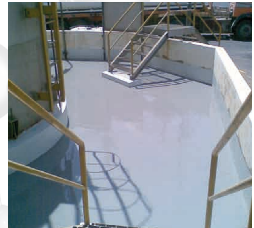
6) Large tank pit for sulfuric acid fabrication
