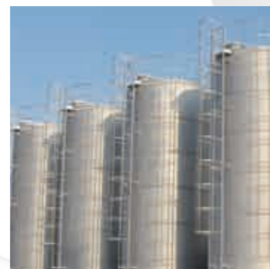
2) Tanks for process water, internal coating
