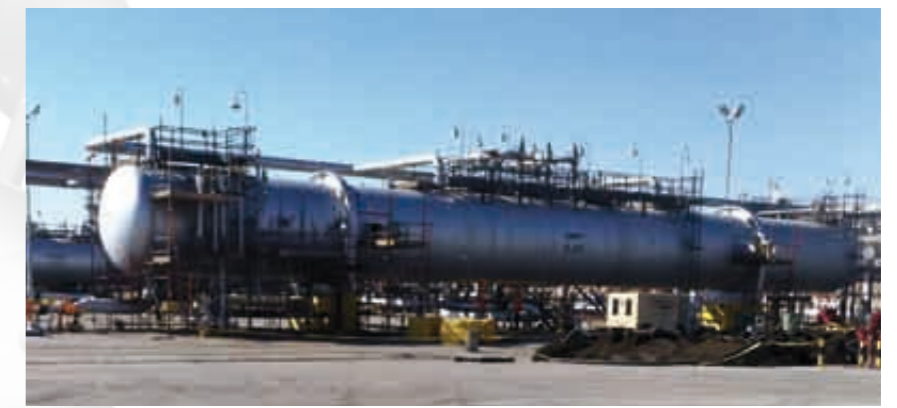
2) Refinery process vessel, internal coating
