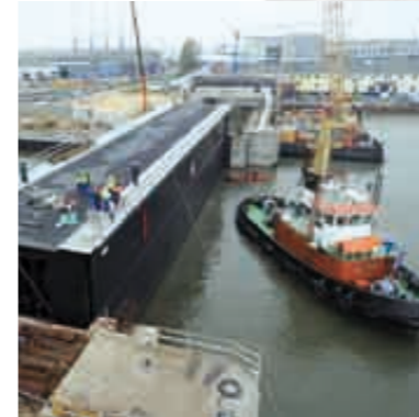
1) Segment of offshore wind energy plant, external coating 2) Lock gate, external coating
