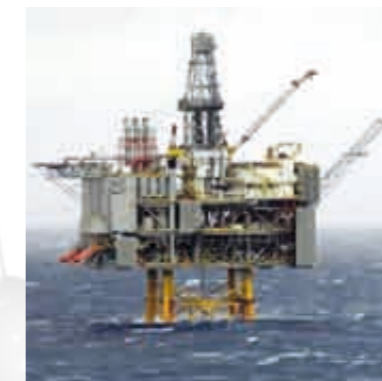
5) Crude oil tanks and separators on offshore platform, internal and external coating
