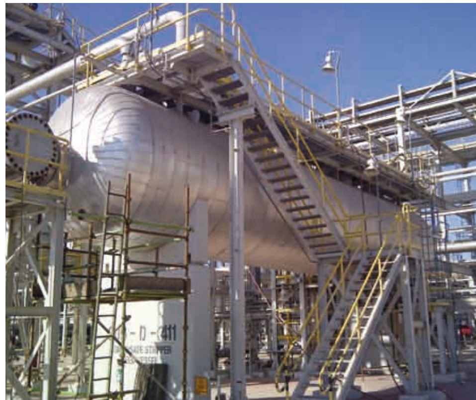
1) Condensate-stripper, gas refinery, internal coating
