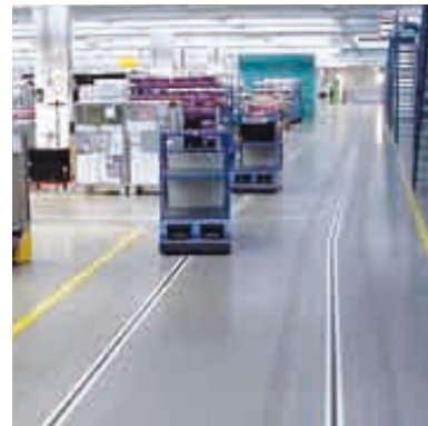
1) Production hall of pharmaceutical industry, chemical resistant floor coating
