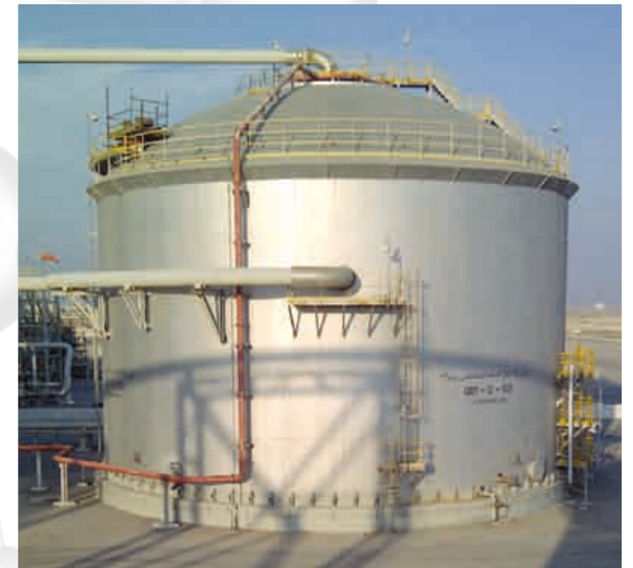
5) Degassing tank, internal coating
