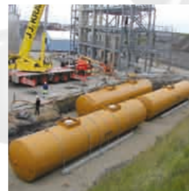
3) Pipeline, internal coating 4) Underground fuel tanks, internal coating
