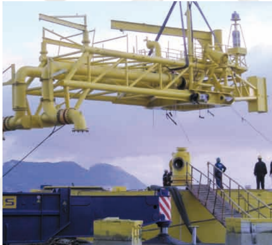
3) Steel construction of singlebuoy mooring system, external coating
