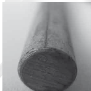
4) Coating with integrated biocide After a month-long test the pickled test rod shows much less corrosion depth. (depth of corrosion cavity 50-80 µm)
