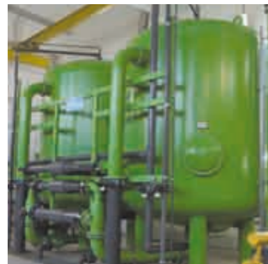
4) Sand filter vessels for drinking water, internal and external coating
