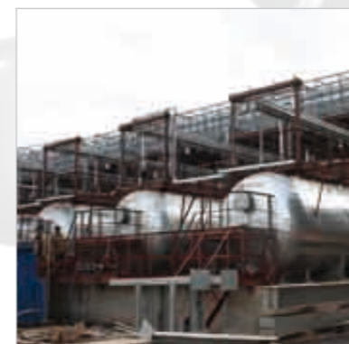
4) Refinery process vessel, internal coating against SRB bacteria
