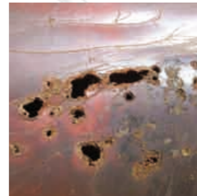
1) Pitting corrosion, induced by anaerobe biocorrosion
