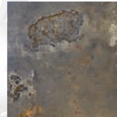
2) Advanced anaerobe corrosion in bottom area of oil tank
