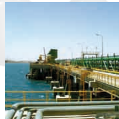
4) Harbour structure, external coating
