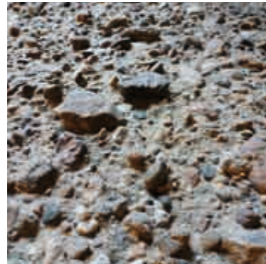
2) Concrete erosions
