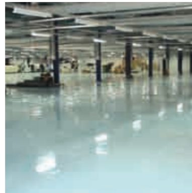
2) Production hall, antistatic flooring system
