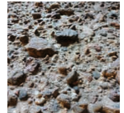
3) Extreme concrete erosions by chemical attack of SRB-produced hydrogen sulfide
