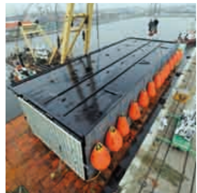
1) Crude oil tanks and separators on offshore platform, internal and external coating 2) Lock gate, external coating
