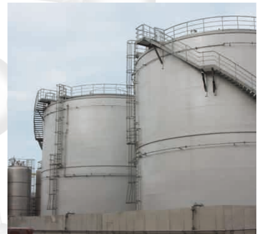
6) Double-walled tanks for ethanol, internal coating and concrete tank pit, external coating
