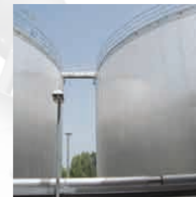
2) Storage tanks of hot fatty acids, internal coating
