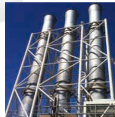
1) Exit flues of chemical plant, internal coating
