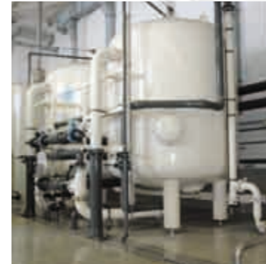
1) Filters for drinking water, internal and external coating
