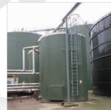
5) Biogas fermenter, internal coating on concrete against SRB bacteria
