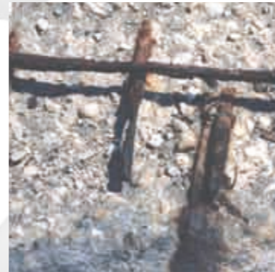
3) Corrosion of steel reinforcement
